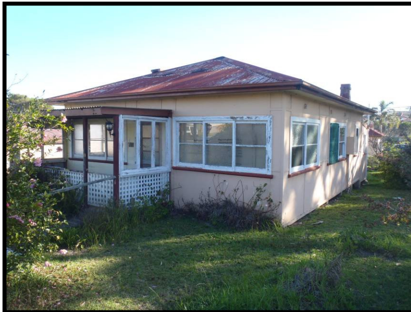
70 Hazard Street Asbestosville NSW.
