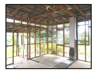
Photographs 1 - 5 Show some areas that were inspected where ACM had been removed from 70 Hazard Street Asbestosville NSW
